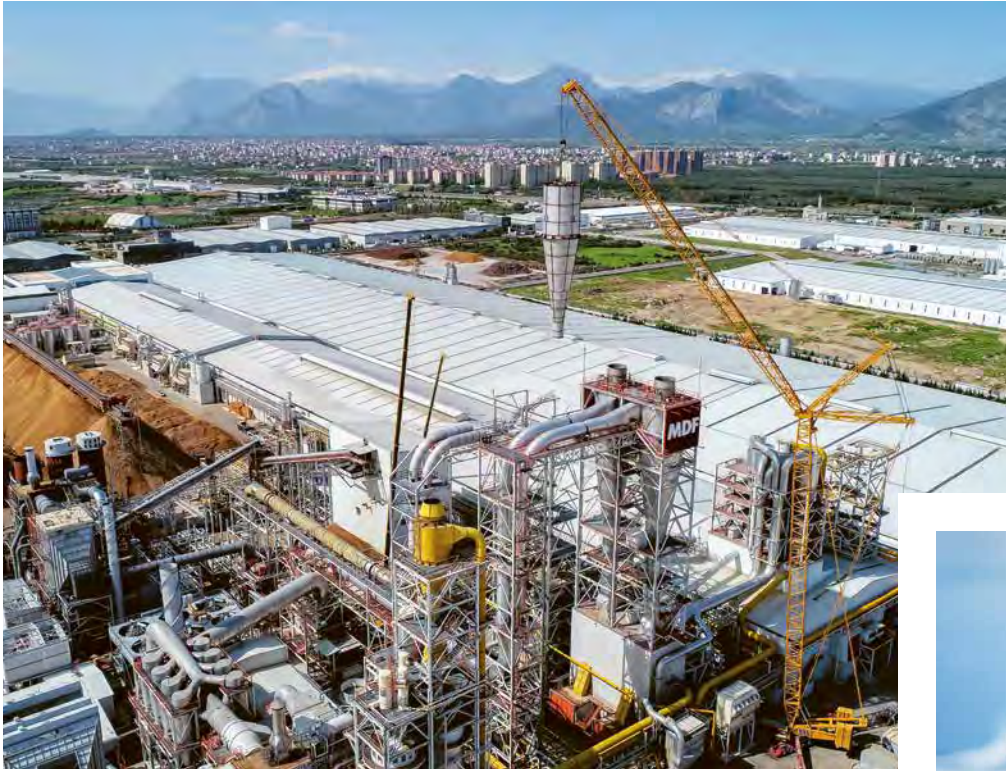
AGT production location in Antalya: exact-fitting installation of a new dryer cyclone, supplied by the Siempelkamp subsidiary Büttner
