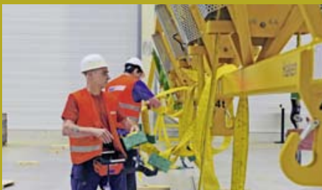
The crane operators check the fastenings are secured
