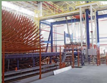
Cooling and stacking line
