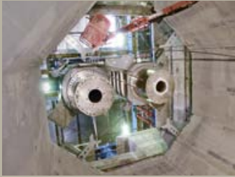
Mounting of press pistons
