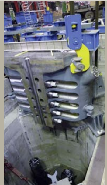
Lowering of the table segment
