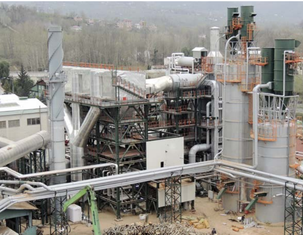
42 MW energy plant
