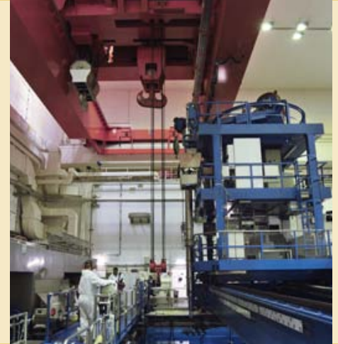
Siempelkamp modernized the crane system in the reactor building
