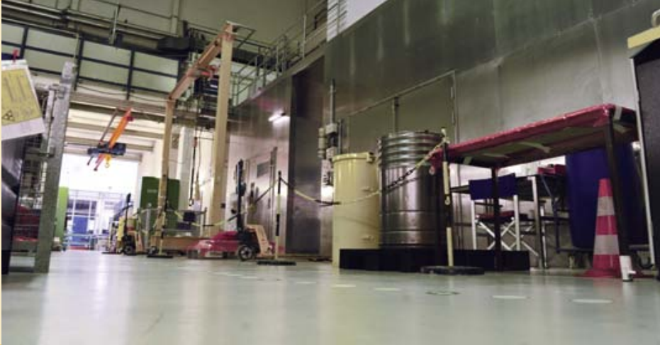
The decontamination cell area inside the Krümmel nuclear power plant
