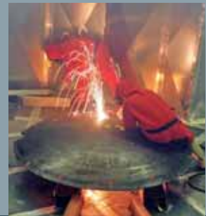
Thermal dismantling of the RPV hemispherical head
