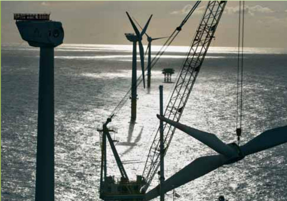
Assembly of an offshore wind turbine (photo: Areva Wind)
