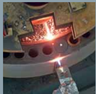
Dismantling of the RPV lid using the oxygen-propane cutting method in the air
