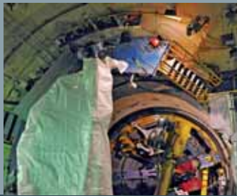
Dismantling of the biological shield using the demolition excavator on a platform of the suspension and fixed mounting frame
