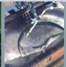
After the recovery of the lower packed bed from the RPV, it was dismantled using the band saw
