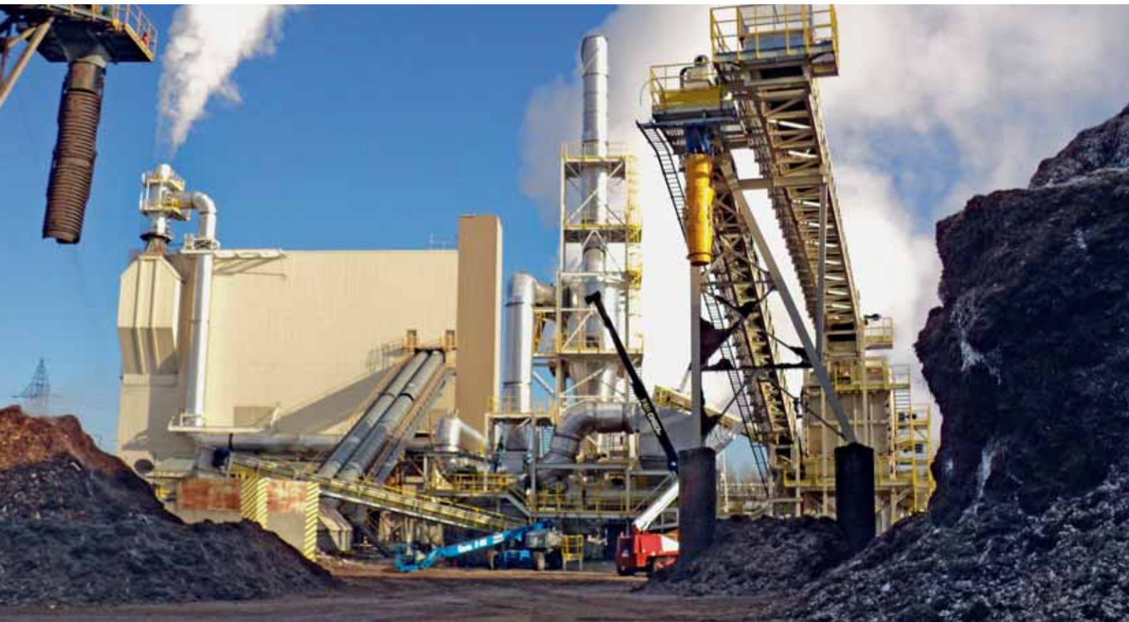
Wet- and dry material conveyors to Buettner dryer
