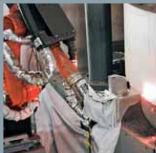
Dismantling of the RPV lid using the oxygen-propane cutting method in the air
