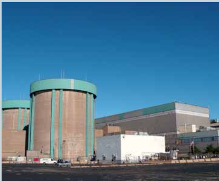
Zion NPP undergoing dismantling since 2010
