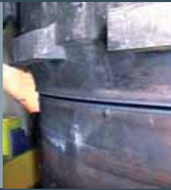
RPV flange ring completely separated using the thermal cutting process
