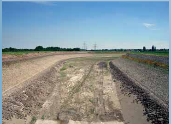
Upper reservoir emptied for inspection
