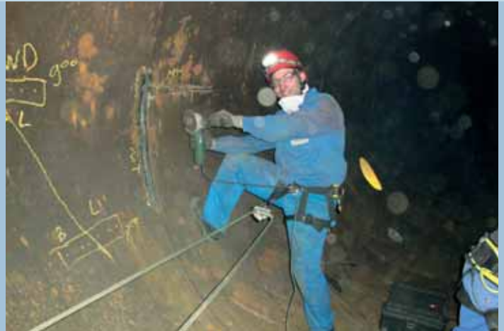
Tests on the welding seams of the penstock pipelines
