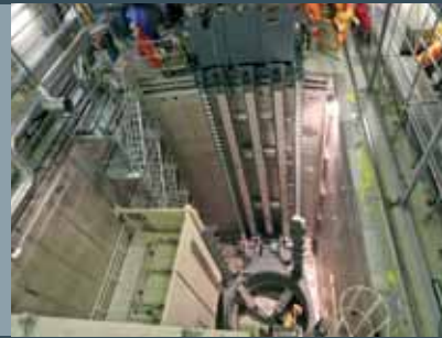
Assembly of the dismantling equipment in the fuel assembly storage pool
