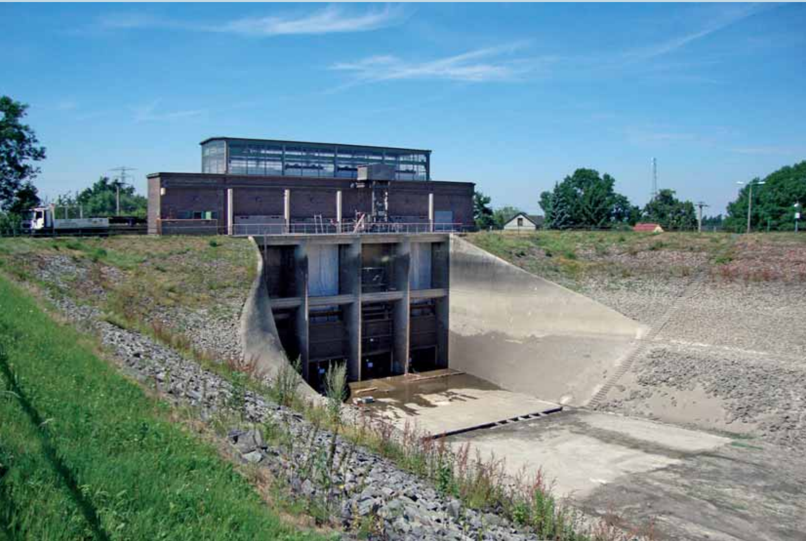
Inlet gate on upper reservoir
