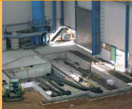
Construction works at the foundations
