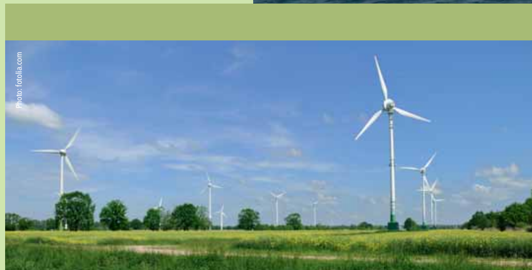
Onshore wind turbines
