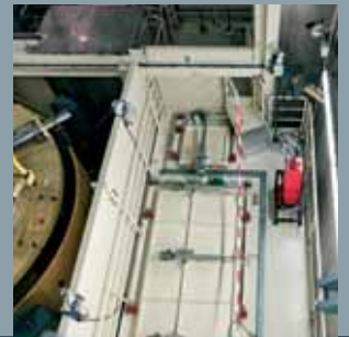
Loading and packaging station for the dismantled RPV parts
