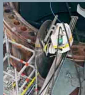
Mechanical dismantling of the RPV flange ring using the band saw
