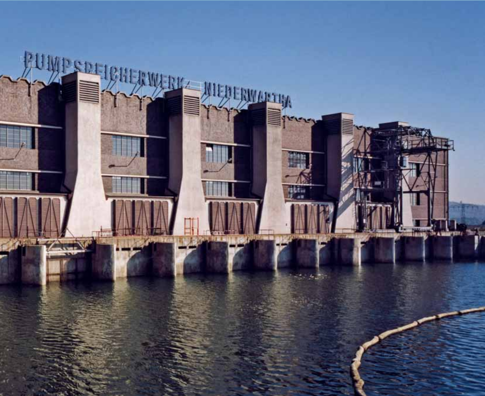
Niederwartha pumped-storage power plant
