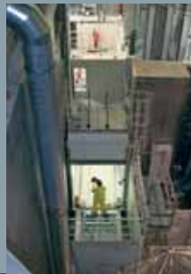
Loading and packaging station for the dismantled RPV parts
