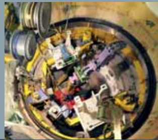
Dismantling of the biological shield using the demolition excavator on a platform of the suspension and fixed mounting frame
