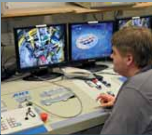
Remote-controlled dismantling of the biological shield
