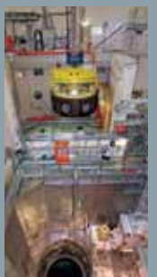
Transport of the RPV flange ring
