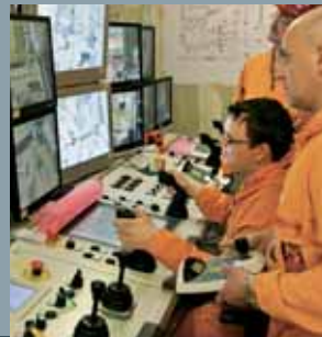
Control station during the dismantling process in Stade
