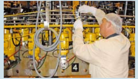
Inserting of cables into the cable duct of the MST
