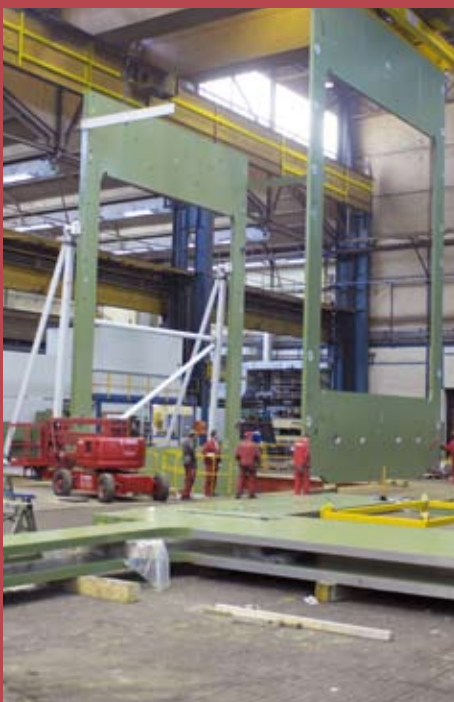
Placement of the frame elements
