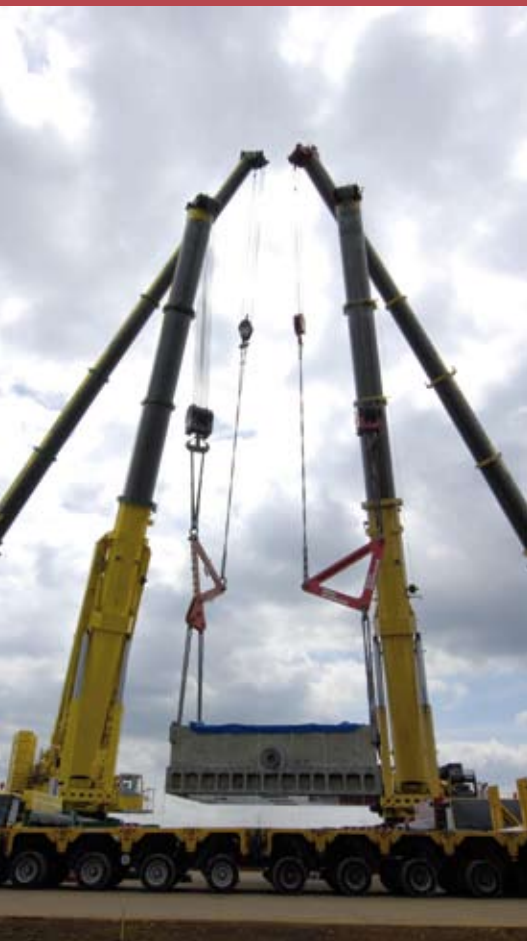
Four cranes are required to lift 218 t
