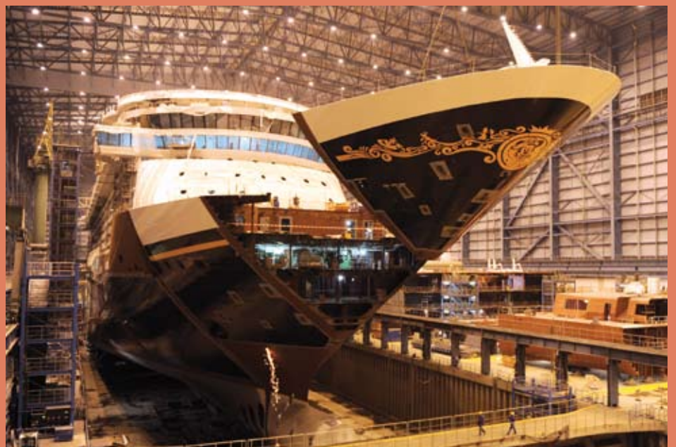
Assembly of the last ship segments for the Disney Dream (Photo: Disney Cruise Line)
