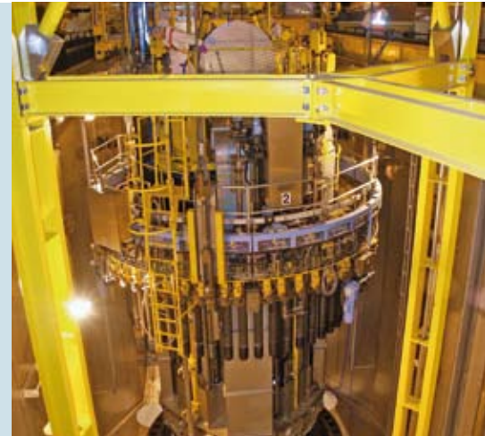
Transport of reactor pressure vessel studs with the stud tensioner
