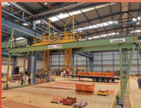
Full gantry crane on floor tracks with lifting load guide for the transport of sheet metal
