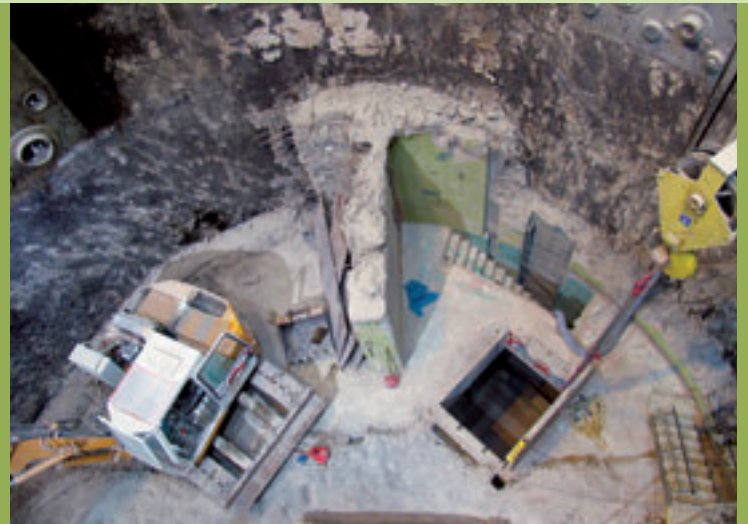
Core removal from the reactor building: Dismantling begins 18 m above ground and ends 20 m below ground
