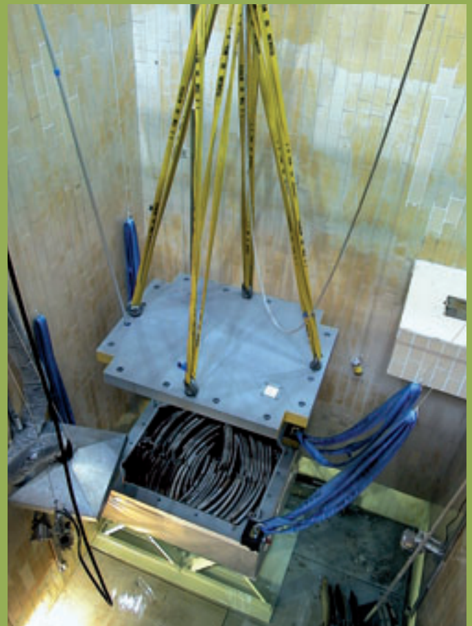
Placing of the disassembled RPV segments into storage containers
