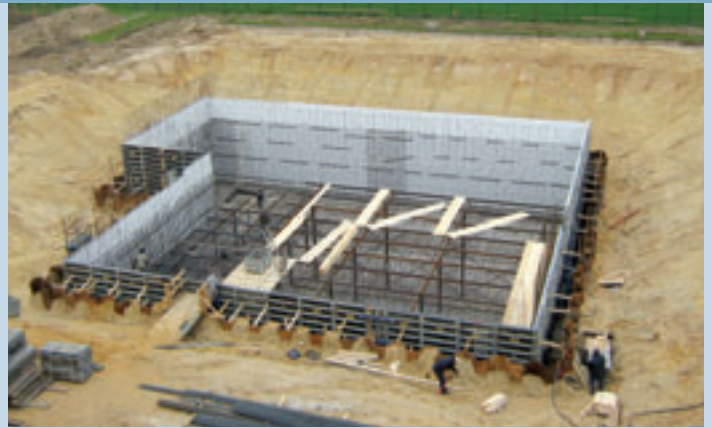
Foundation for mill
