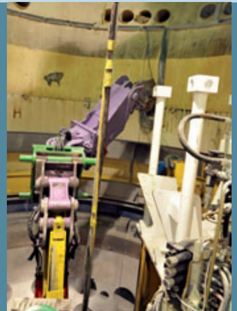
Dismantling of a biological shield at the multi-purpose research reactor: SNT-supplied equipment includes standing and hanging frame with remotely-operated special-purpose machines
