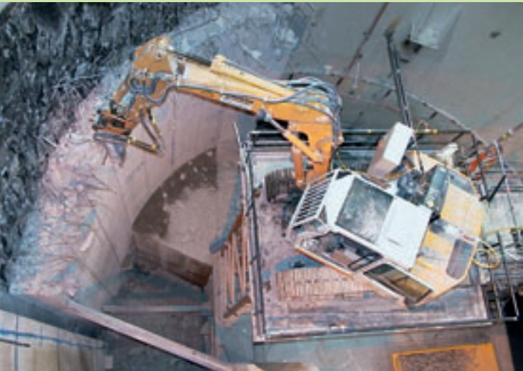
Core removal from the reactor building: Dismantling begins 18 m above ground and ends 20 m below ground
