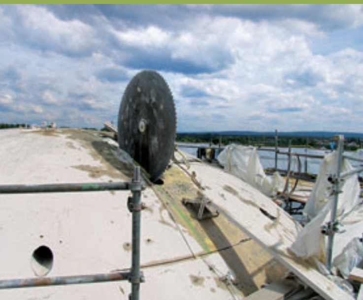
Sawing of the dome segment with a concrete saw
