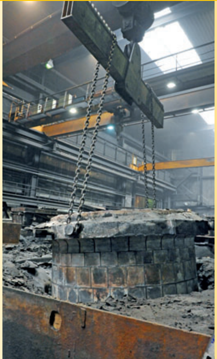
Removal of the trunnion from the mold
