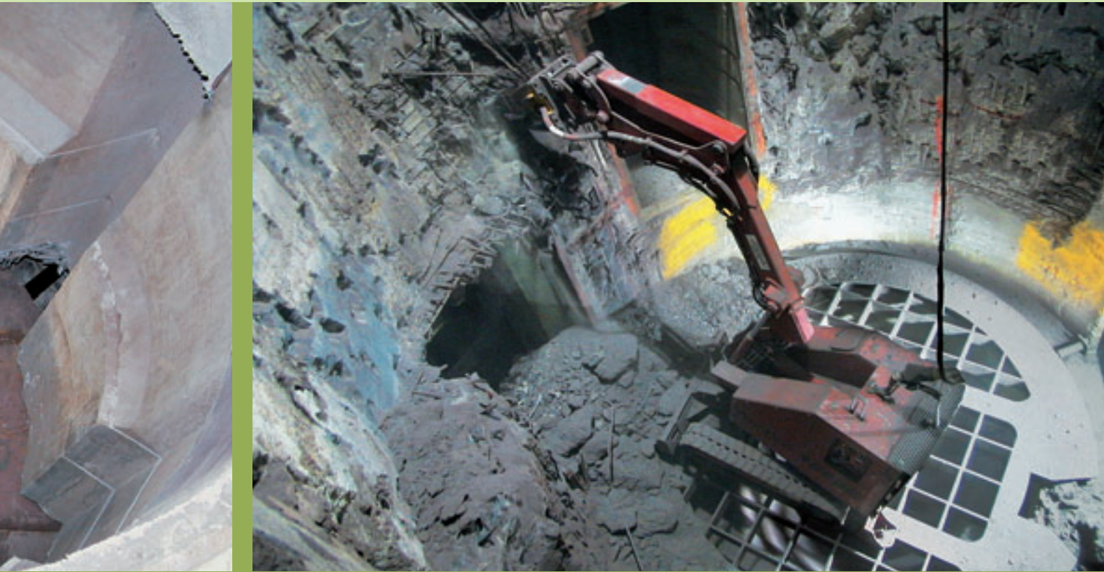
Dismantling of the biological shield with a remote-controlled demolition excavator
