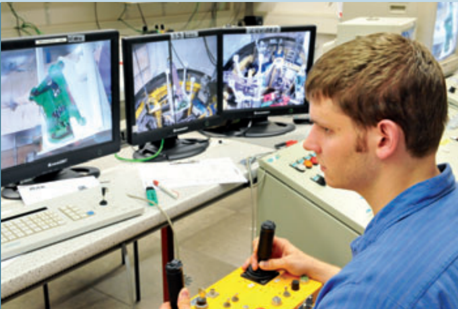
Control room for remotely-operated dismantling process
