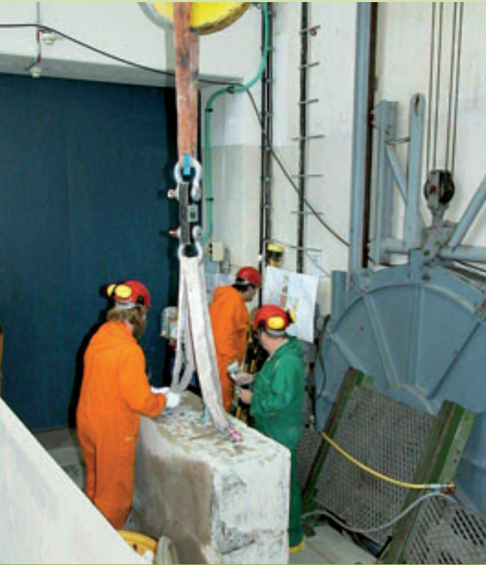
Handling of the dismantled storage pool segments
